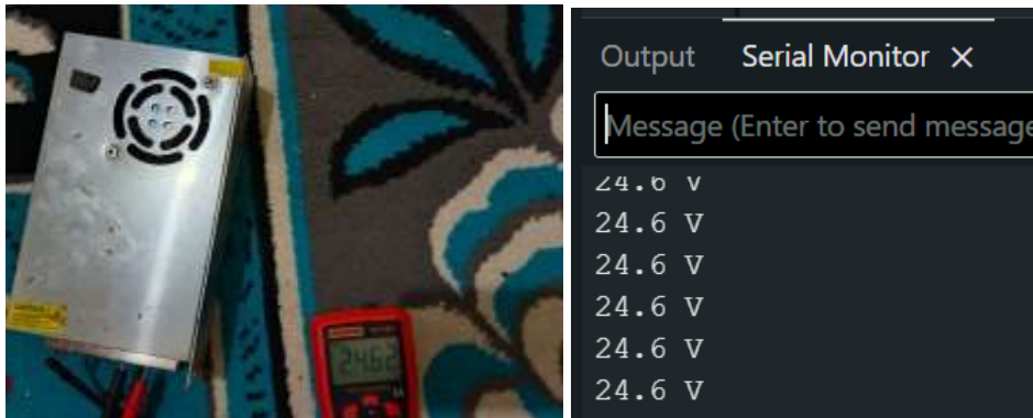
Gambar 4. 9 Pengujian Power Supply
