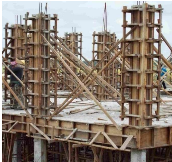
Gambar 4. 2 Bekisting Plywood
